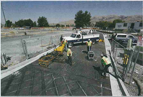
Left: Top Grade Construction processes decorative asphalt in Milpitas, CA. (All photos courtesy of Top Grade Construction)
